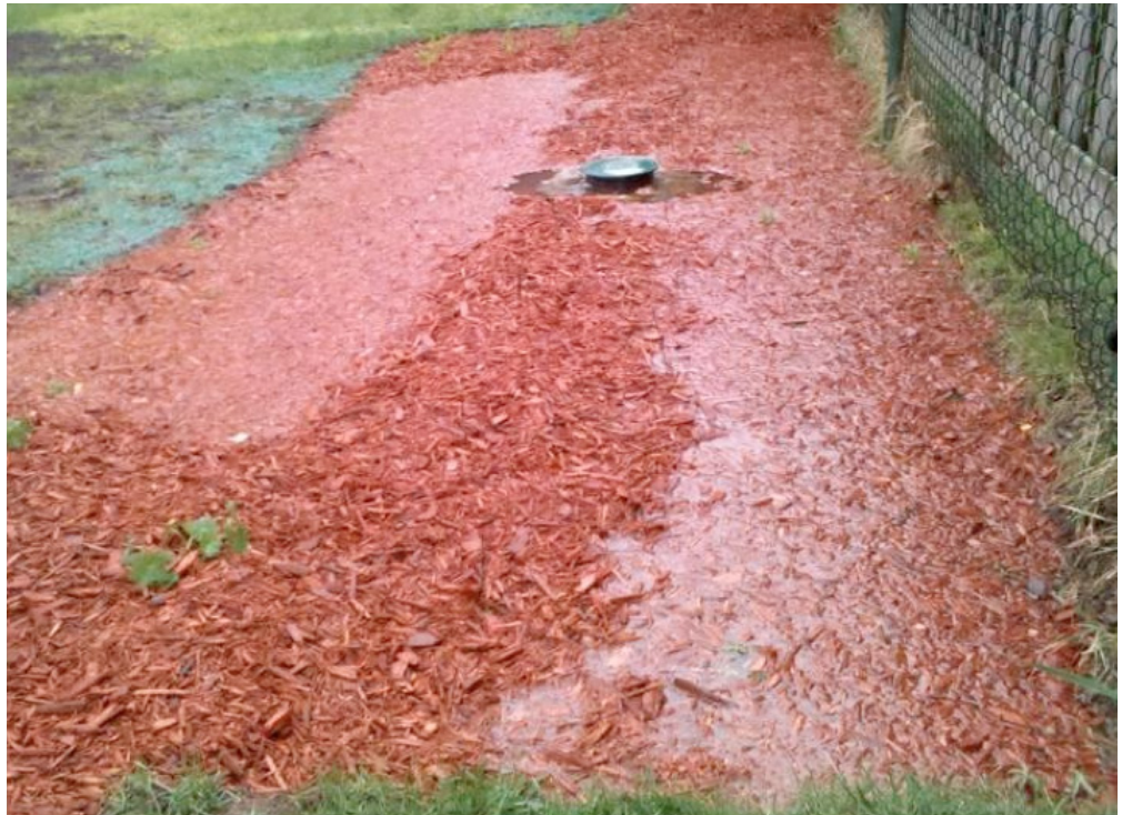
Figure 15: This pop-up emitter releases water into the rain garden.
