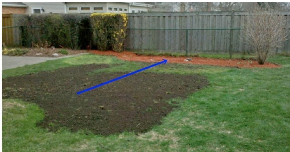
Figure 16: Grading water into the rain garden.
