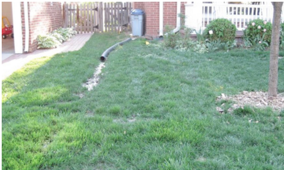
Figure 8: Sump pump outlet causing standing water issues.
