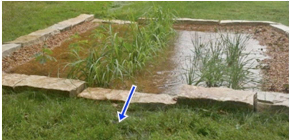
Figure 18: The installer and homeowner must decide where overflow water goes so that it has safe path off the property.
