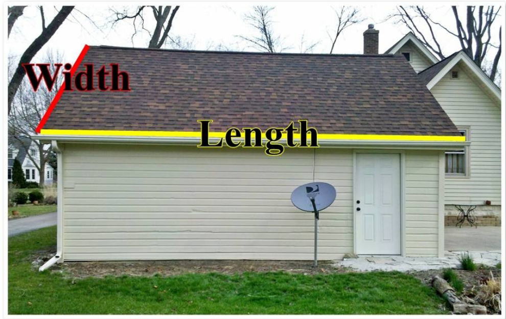
Figure 4: Determining the surface area of the roof.
